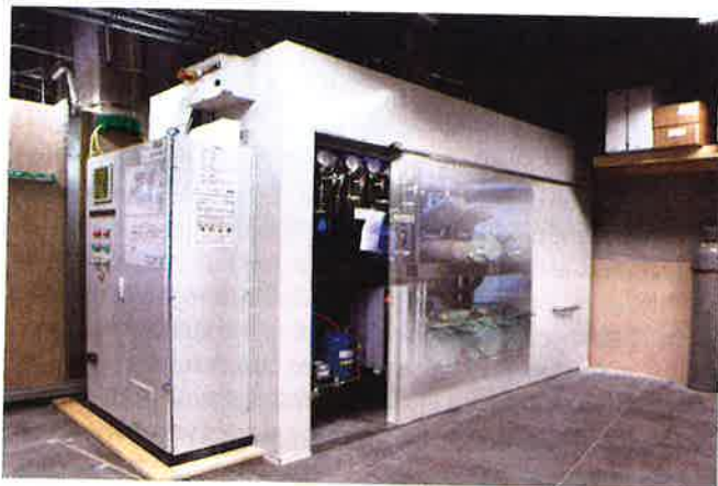
Figure 7: The CO 2 booster system
