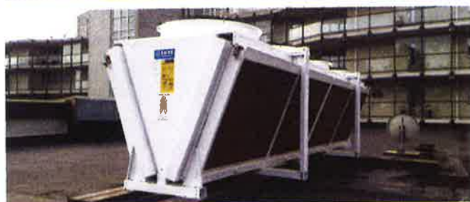
Figure 4: Gas cooler (with adiabatic panels and EC motors)
